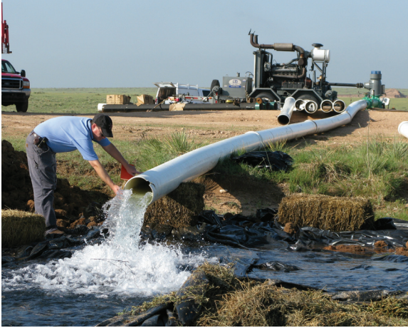
Prototype supply wells demonstrated production capacities ranging from 850 to 1,140 gpm.
