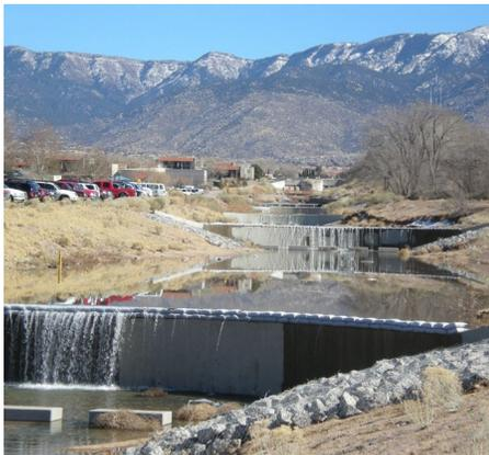
This Albuquerque Bernalillo County Water Utility Authority (ABCWUA) Bear Canyon Aquifer Recharge project is **the first to obtain a permit for full-scale operation in New Mexico**. The project involves releasing surface water into an arroyo channel and monitoring it as it moves through the 500-foot-thick vadose zone profile.
